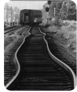
(Example 10.3) Thermal expansion: The extreme heat of a July day in Asbury Park, New Jersey, caused these railroad tracks to buckle.
