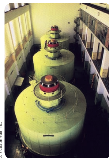
Turbines turn electric generators at a hydroelectric power plant.
